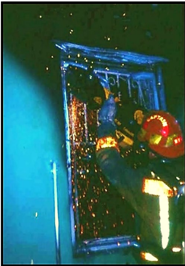
CAPTAIN BILL GUSTIN WORKING ON SOFTENING UP THE STRUCTURE AS HE CUTS BARS OFF A WINDOW
